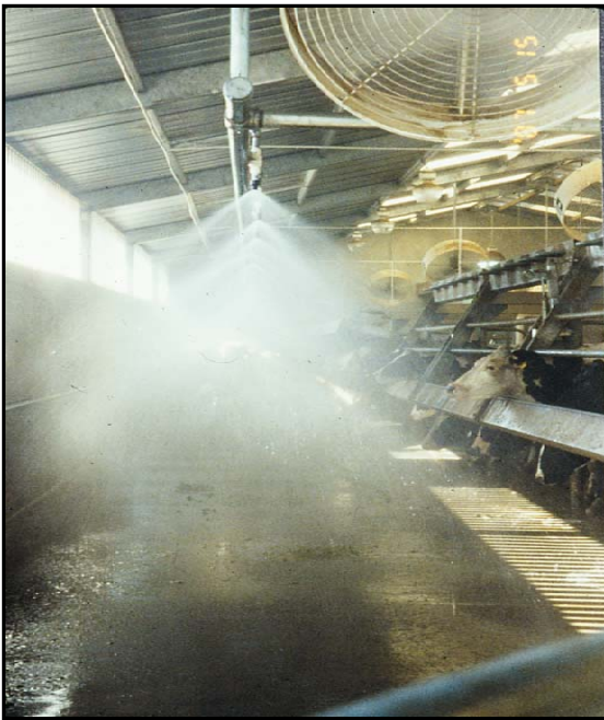
Large nozzles on exit platform
